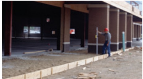
Forms and Footings
